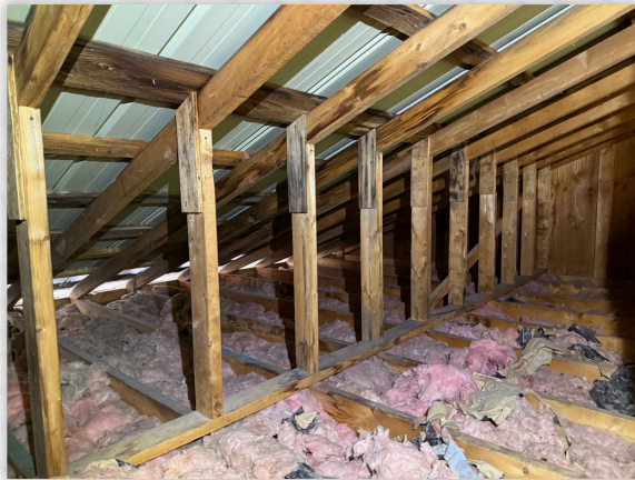
Style 1: Older "Homemade" Trusses
